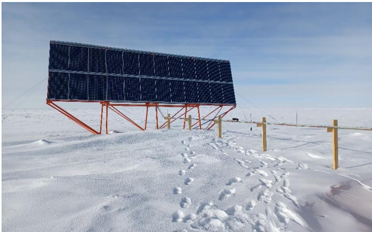
Figure 1: Solar panels structure at Concordia. (Credit: IPEV)
