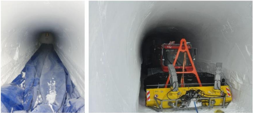
Figure 1: Internal views of the garage, with the deflated balloon still on the floor (left) and the vehicles parked in the cave for the winter. (Credit: ENEA/PNRA)
