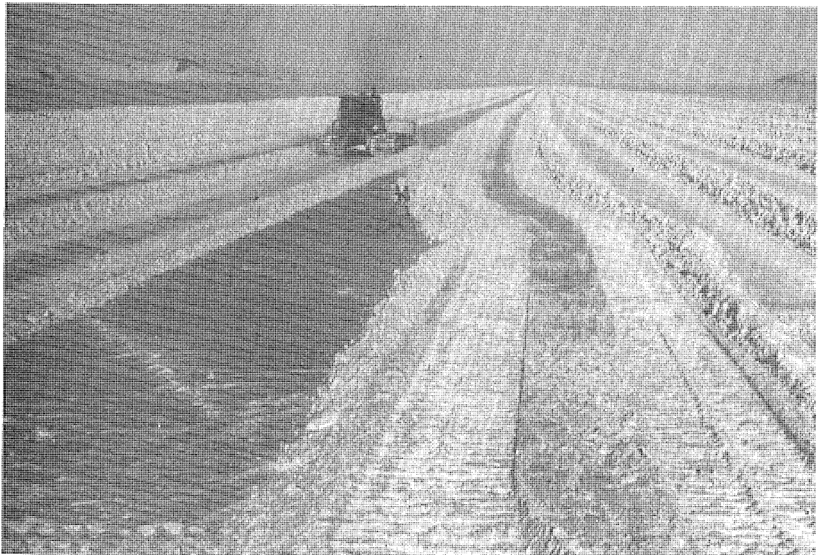
Figure 10. Bulldozer stripping and windrowing snow on runway site.
