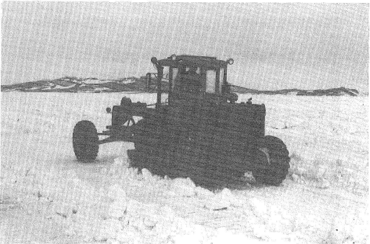
Figure 11. Grader used to distribute windrows.
