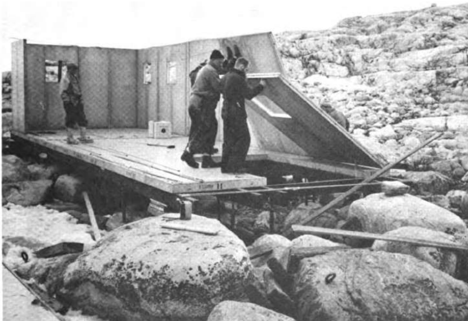
Erection of walls. Note tie-rods laid out ready for insertion.
