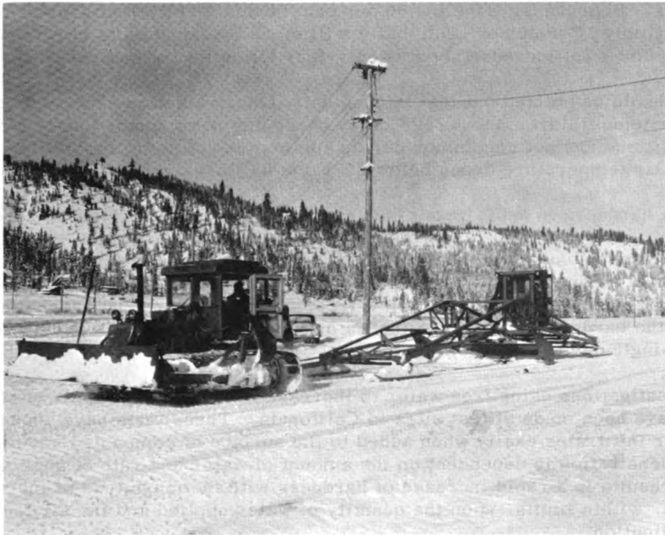
Figure 5. The Navy snow tractor towing the Model 40 snow plane.
