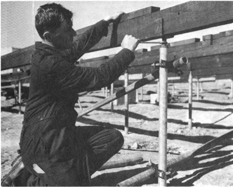
Pipe foundations and bearers showing fine adjustment of forked reveal pins.
