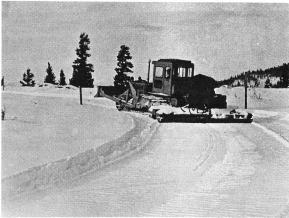
Figure 9. Smoothing snow road with snow finishing drag.
