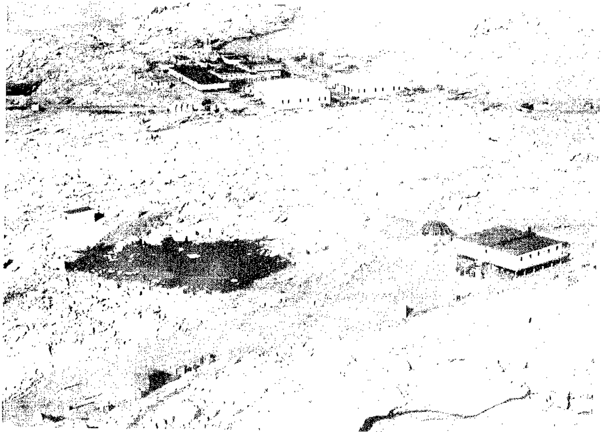
Fig. 2 View of Terra Nova Bay Station
