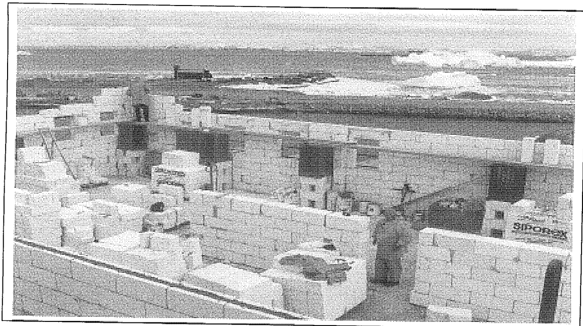
Figure 4: Generation 5 "Siporex" building under construction
