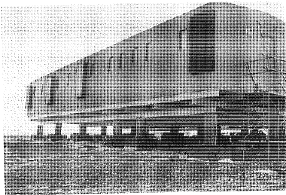
Fig.4 Solar collectors set on the wall
