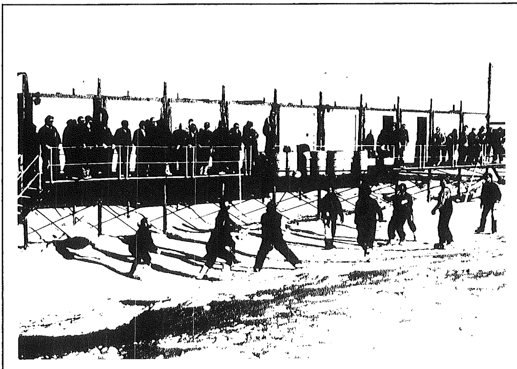
Figure 1 The temporary construction base
