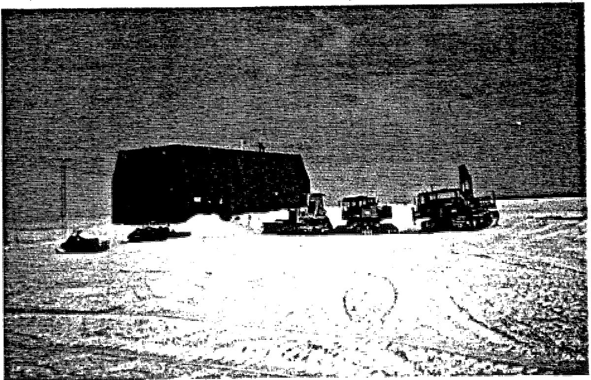
GARAGE/WORKSHOP IMMEDIATELY AFTER CONSTRUCTION FEBRUARY 1993
