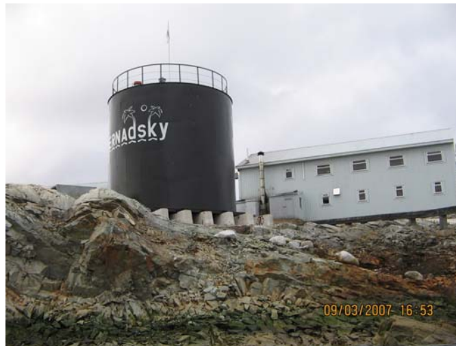
Figure 1: Vernadsky Station showing fuel reservoir installed in 2007
